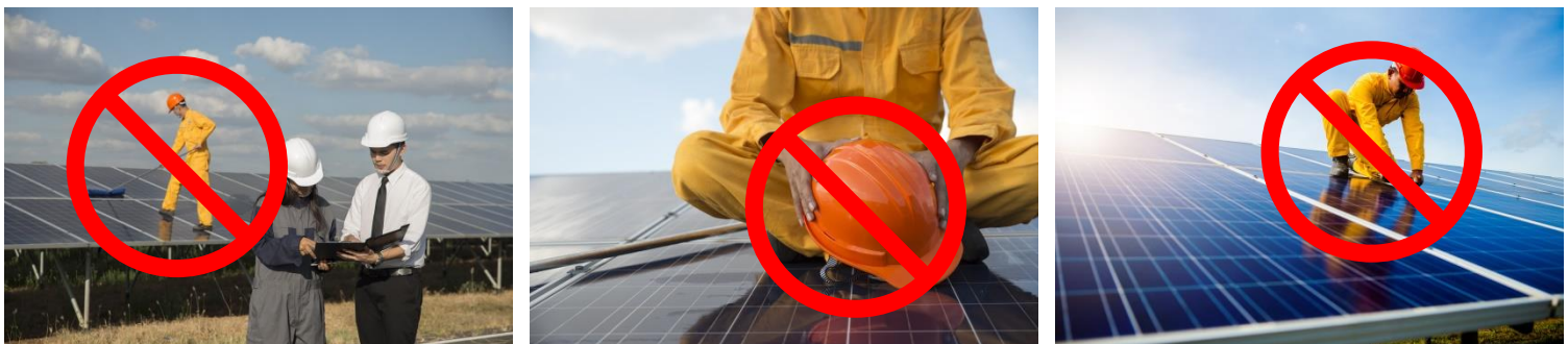
Figure 1: Wrong methods of installing a solar PV module
